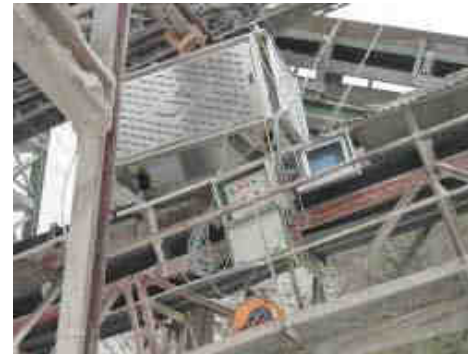
A laser-induced fluorescence (LIF) analyzer.
